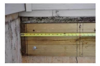
Lay out your bolt locations using a tape measure and construction pencil. Bolt patterns will vary depending on joist length. Bolts should be staggered between joists and located 2" from the top and bottom of the ledger board.
