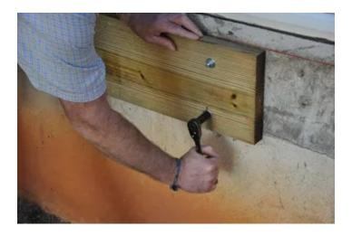
Hand tighten the bolts using a ratchet. Do not over tighten.
