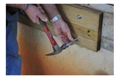
Install two bolts at the end of each ledger board. Hammer the sleeve anchor through the ledger board into the concrete wall.
