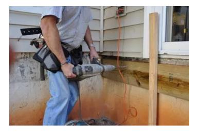
Temporarily secure the ledger board to the correct location against the concrete wall using concrete screws or temporary supports. Use a wood bit to drill ½" pilot holes through the ledger board. Next, use a concrete bit to drill into the concrete wall.
